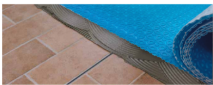
Ceramic flooring with expansion joints
