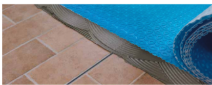
Ceramic flooring with expansion joints
